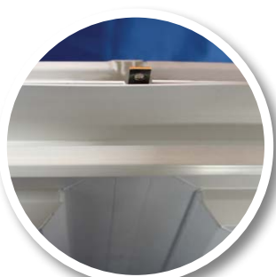
Drip Cap with Bracket to attach mullion to rough opening.
